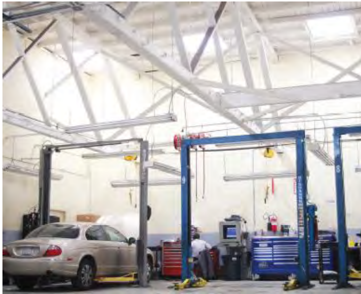
Dealership Suntracker Installation
